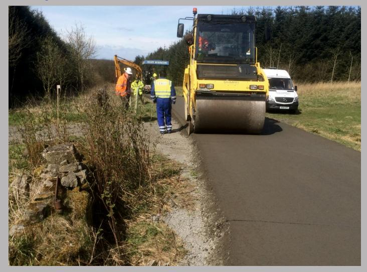
The finishing touches to a road surface laid within 6hrs of starting. Light vehicle use is achievable within a few hours with heavy traffic running on this surface the next day. The running surface has a similar finish to that of tar macadam. The areas can be varied in size as the jointing of the material is not effected in any way. All areas require to be laid on a regular even gradient. Similar to tar the product is only laid when dry conditions above are in place.
